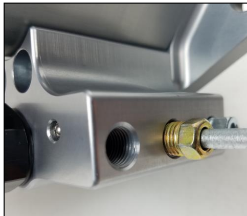
Figure 6: Hard Line Installation
